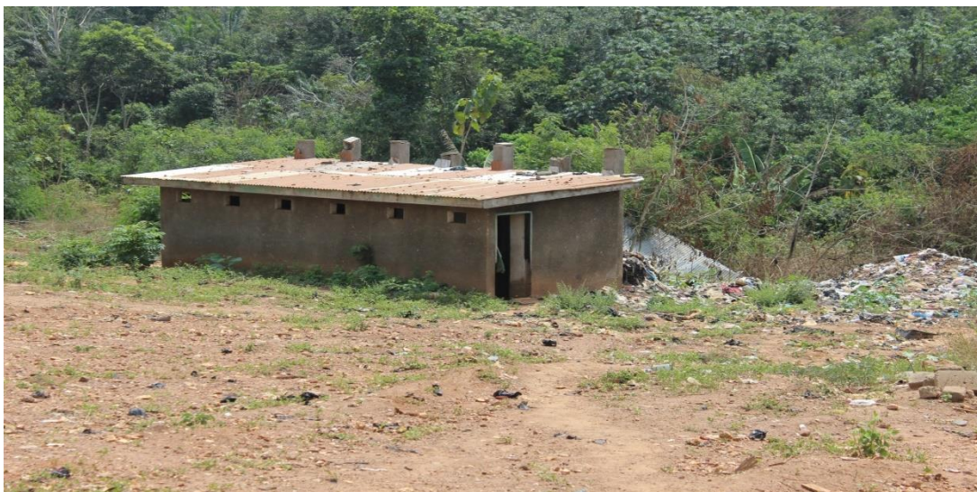
Toilet facility at Obenemase, adjacent to garbage disposal site; March 2017
