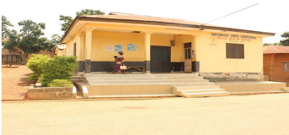
CHPS facility at Obenemase; March 2017
